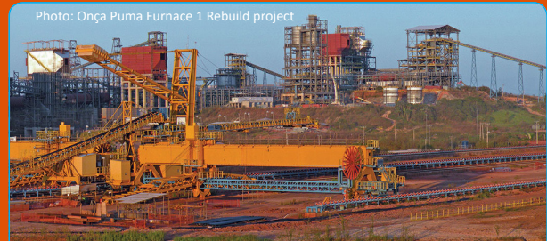
Photo: Onça Puma Furnace 1 Rebuild project
